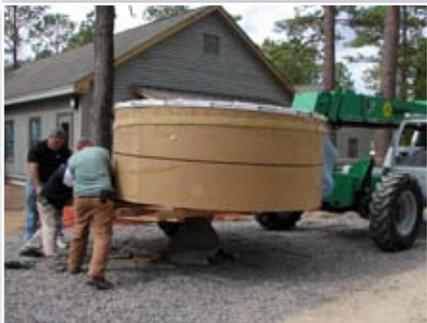
*The tank arrives and is carried to an opening left in the building for this purpose.*
