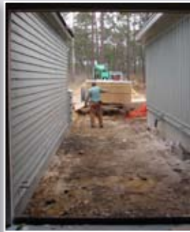
But will the 8 ft diameter tank fit through the opening?
