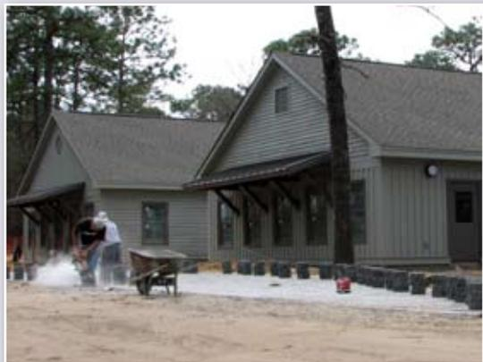
Permeable pavers were installed in the bus drop-off area and walkways next to the Discovery Center. These pavers provide a sturdy surface for car and foot traffic and can reduce or eliminate stormwater runoff. Under the pavers, an open-graded bedding layer and aggregate base allow stormwater to filter through, trapping pollutants on the way. The water then infiltrates into the ground where it is purified and eventually recharges ground water sources.
