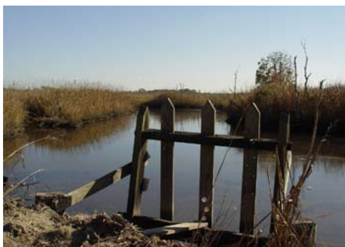
Rice field trunks, such as this, control the water flow between tidal creeks or rivers and the impoundments. (Photo courtesy, R. Szivak)
