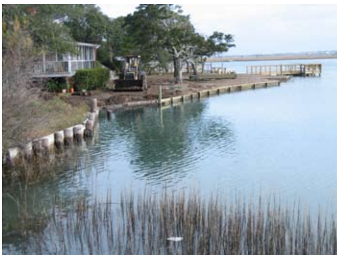
A failing bulkhead allows sediment to wash directly into a tidal creek in coastal South Carolina. (Photo courtesy, J. Pollack)
