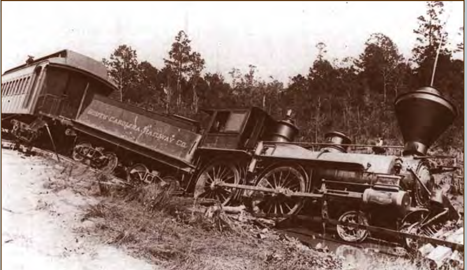
Train washed from tracks by a four-foot high wall of water when the Charleston earthquake burst the mill dam at Langley Pond near Aiken, SC.
